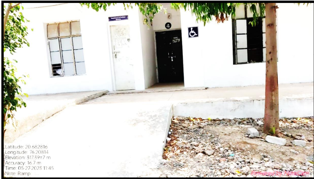
Divyangjan- Friendly, Barrier-Free Environment: Ramp-3 For Block B.
