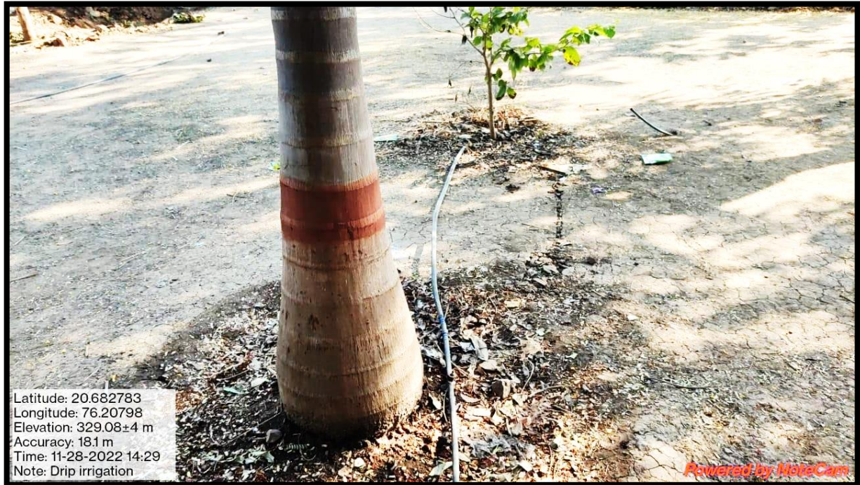
Water Distribution for Plants by Drip Irrigation System.
